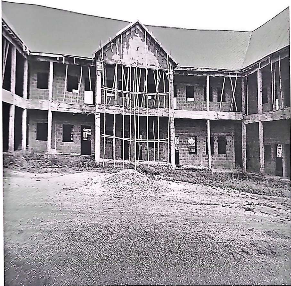
School Block at Ezzikwo Road Urban Primary School Abakaliki, Ebonyi State
