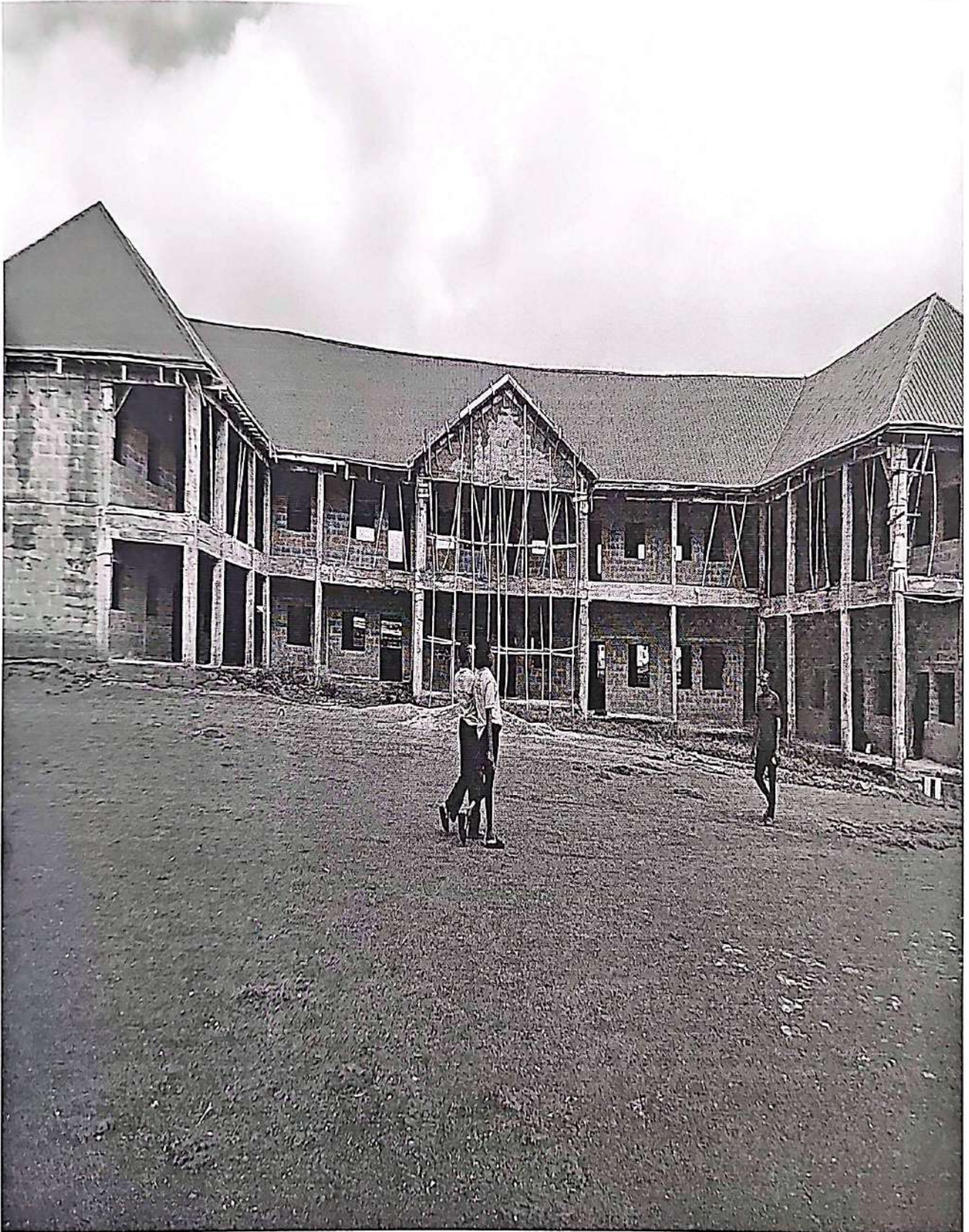
School Block at Ezzikwo Road Urban Primary School Abakaliki, Ebonyi State
